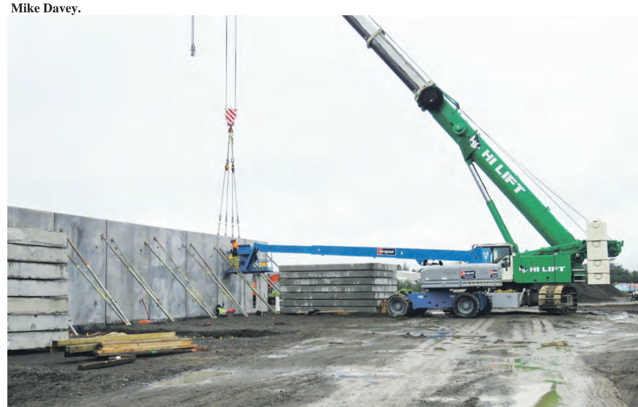
The bin walls for the giant New Plymouth store are placed in a row. Each concrete panel weighs 22 tonnes (including eight tonne of steel) and there are 321 to erect. That's heavier than the Statue of Liberty.
